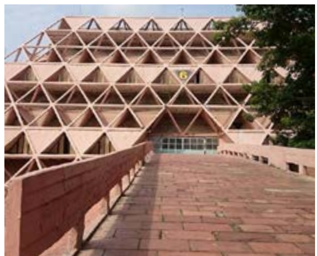
The Hall of Nations Complex before demolition Image source: Kiran Joshi
