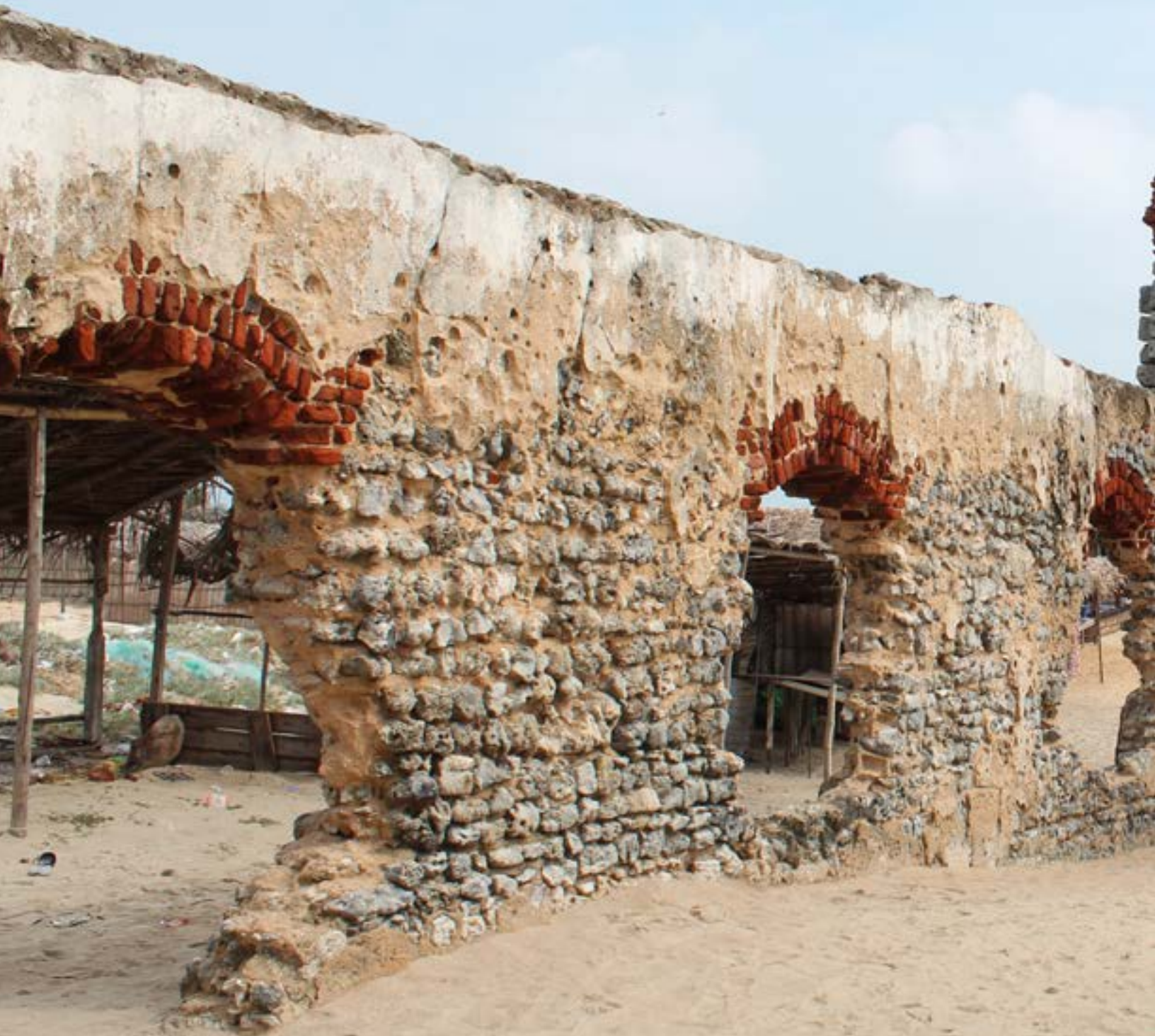
Ruins of church built of coral and brick, Dhanushkodi, Tamilnadu, image by Samhitha Polamuri
