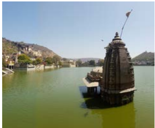
Half-submerged Temple dedicated to Lord Varuna- the vedic god of water- at Nawal Sagar, Bundi_PSingh
